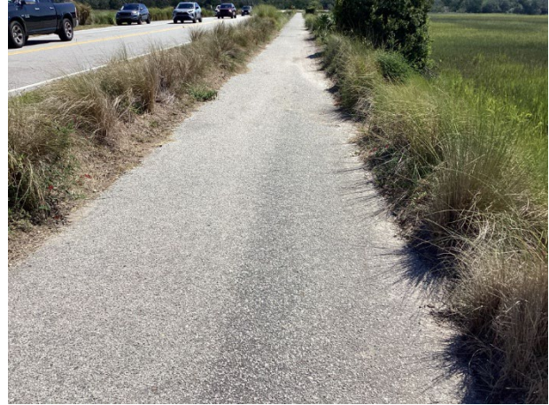
Asphalt pavement walking path
