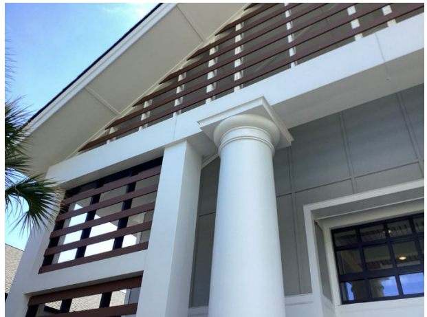
Fiber cement siding overview
