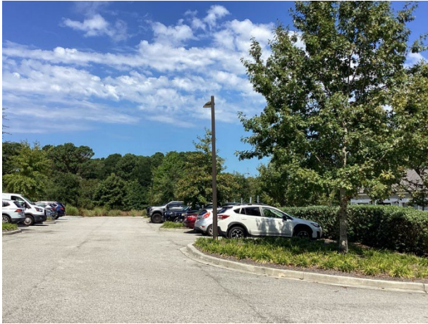
Light pole and fixture
