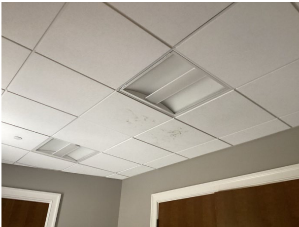
Acoustical ceiling tiles overview
