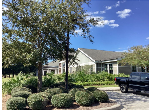
Light pole and fixture
