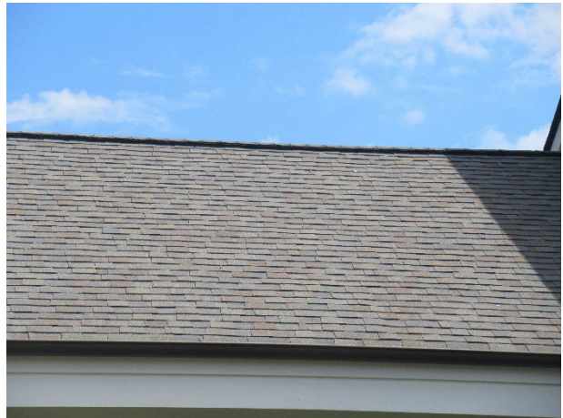
Asphalt shingle roof overview
