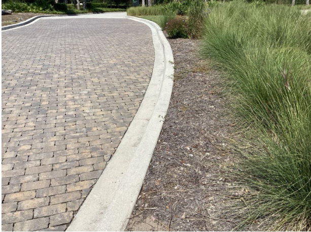
Concrete curb and gutter
