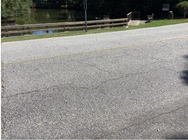
Pavement cracks
