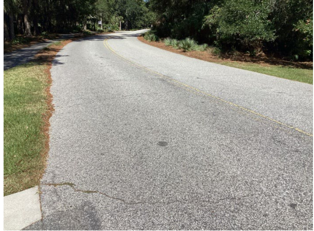
Pavement cracks
