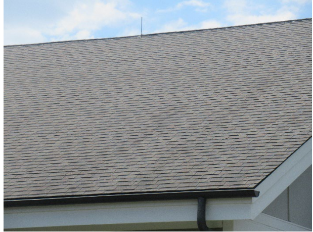
Asphalt shingle roof overview
