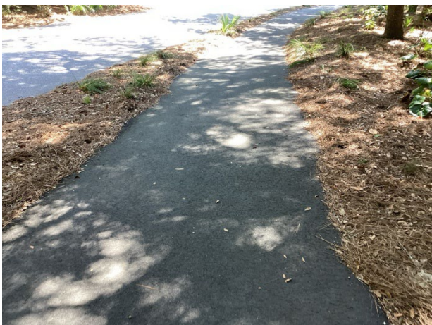
Asphalt pavement walking path
