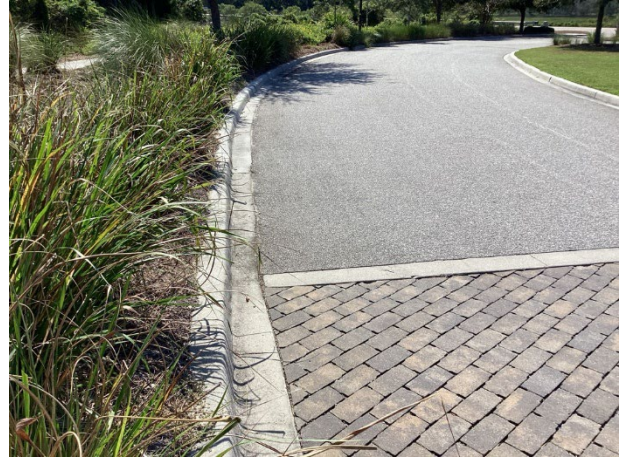
Concrete curb and gutter
