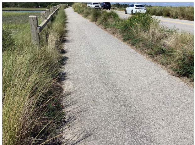
Asphalt pavement walking path
