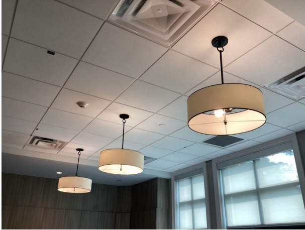
Acoustical ceiling tiles overview
