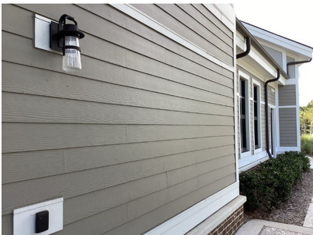
Fiber cement siding overview
