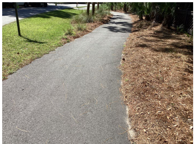
Asphalt pavement walking path
