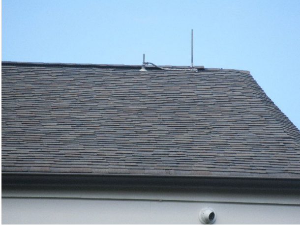
Asphalt shingle roof overview
