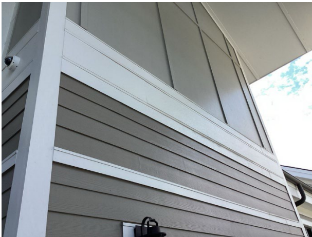
Fiber cement siding overview
