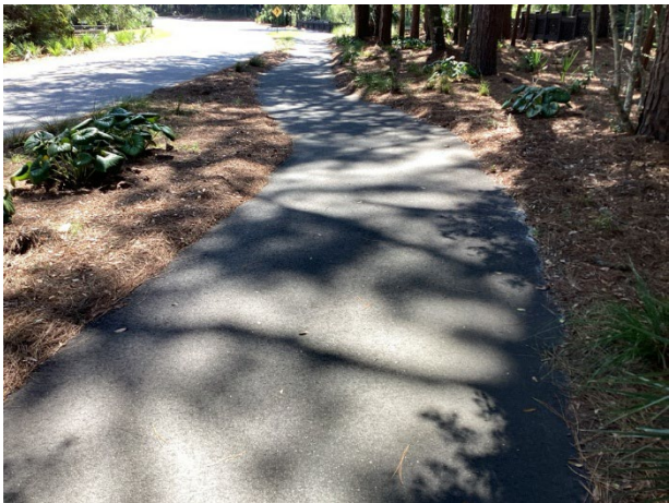
Asphalt pavement walking path
