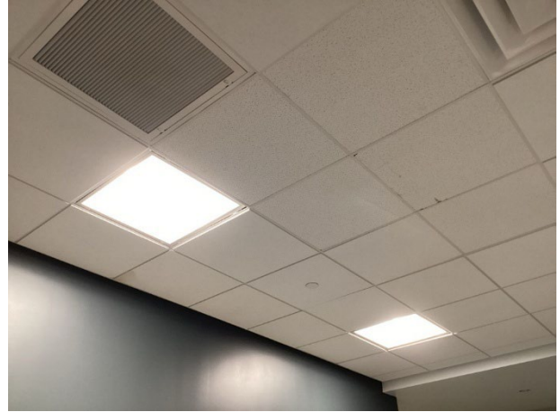
Acoustical ceiling tiles overview
