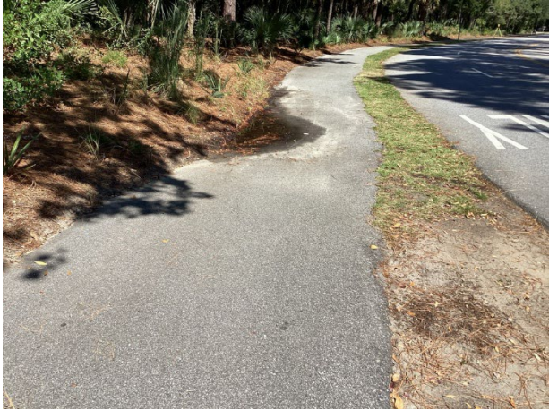
Asphalt pavement walking path
