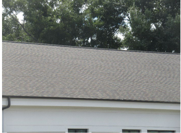
Asphalt shingle roof overview
