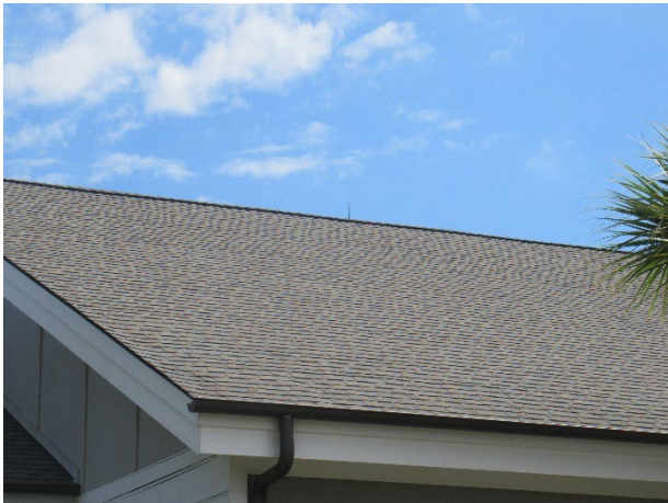
Asphalt shingle roof overview
