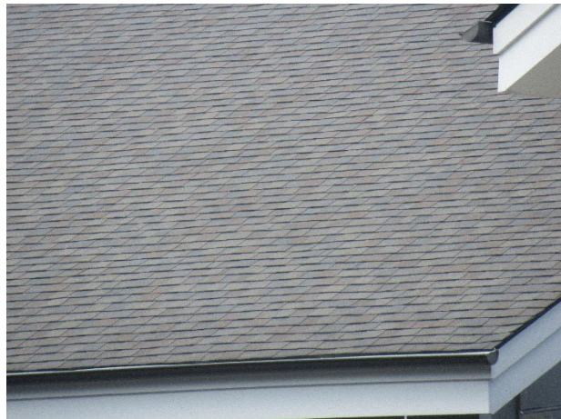
Asphalt shingle roof overview
