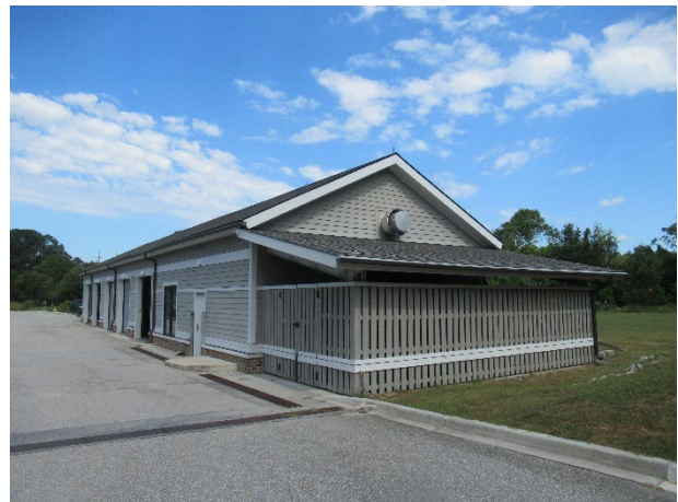
Maintenance building overview
