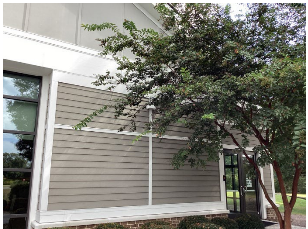
Fiber cement siding overview
