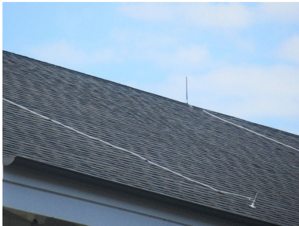
Asphalt shingle roof overview
