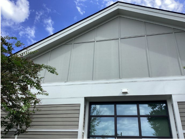
Fiber cement siding overview
