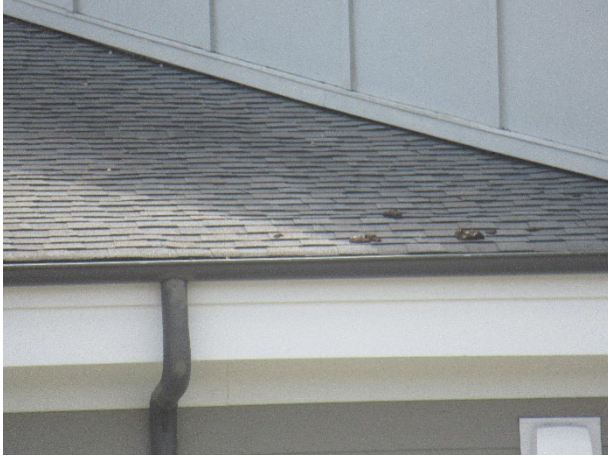
Asphalt shingle roof overview – Note minor debris accumulation
