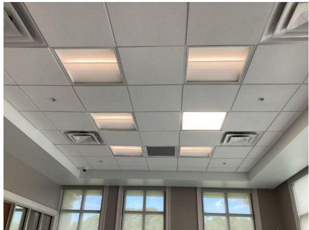
Acoustical ceiling tiles overview
