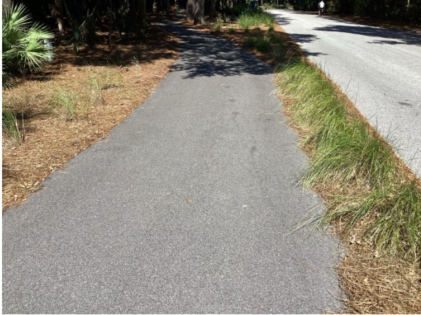
Asphalt pavement walking path
