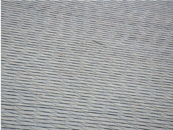
Asphalt shingle roof overview
