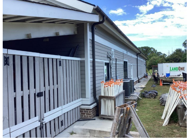
Fiber cement siding overview
