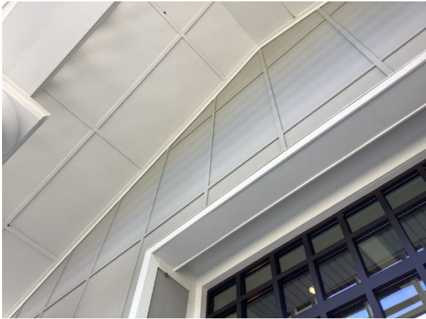
Fiber cement siding overview
