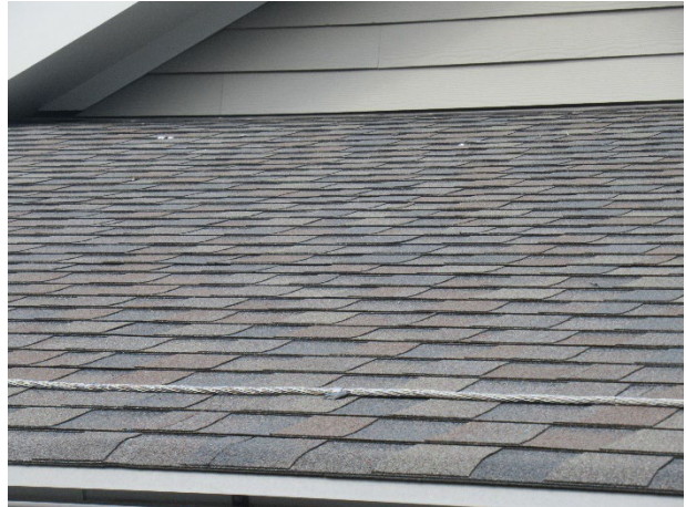
Asphalt shingle roof overview
