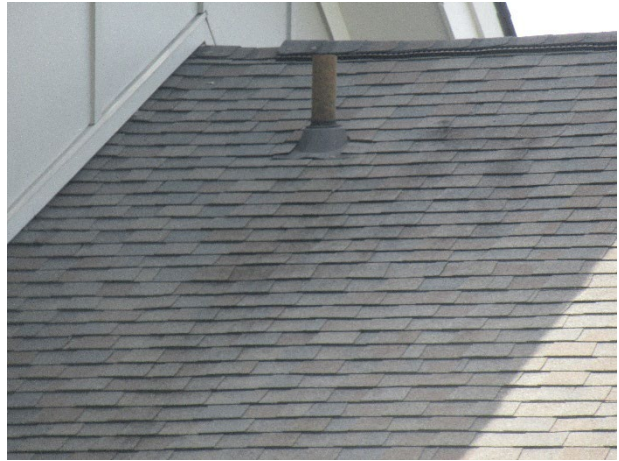
Asphalt shingle roof overview – Note minor stains
