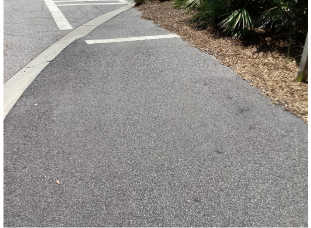
Asphalt pavement walking path
