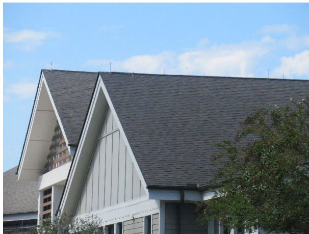
Asphalt shingle roof overview
