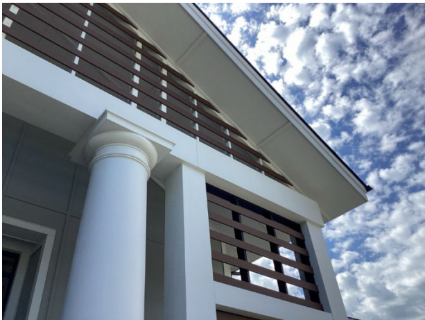
Fiber cement siding overview
