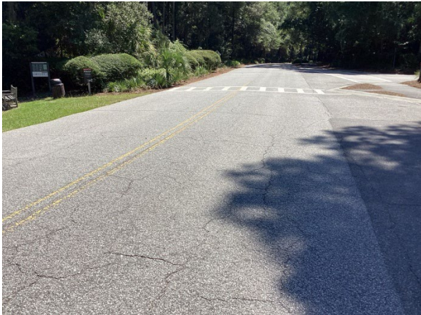
Pavement cracks
