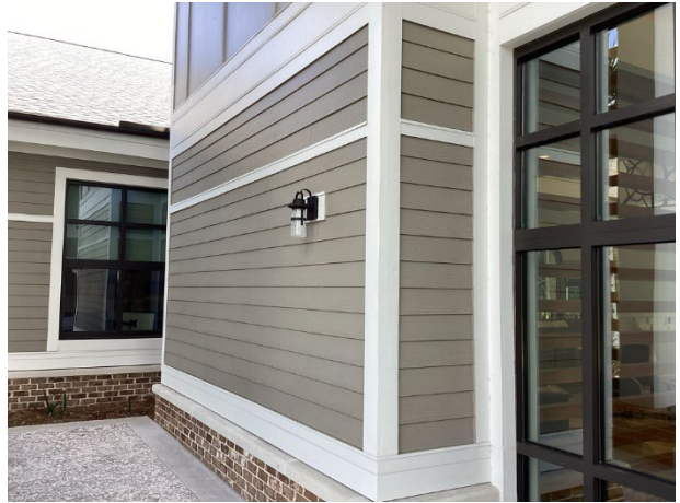
Fiber cement siding overview
