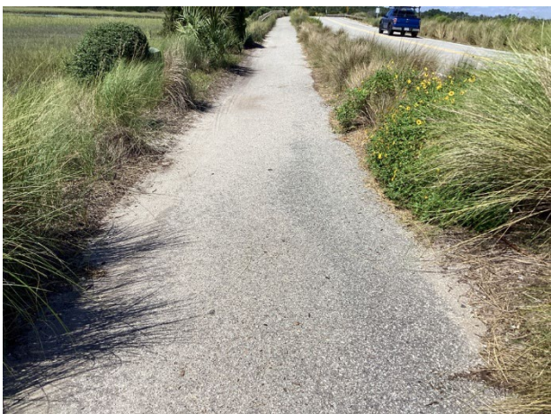
Asphalt pavement walking path
