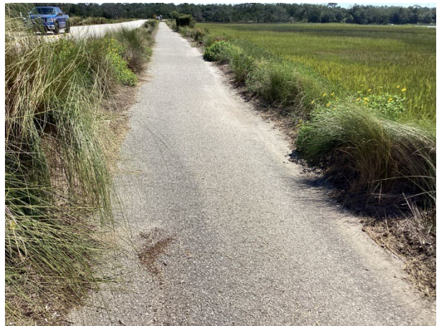
Asphalt pavement walking path
